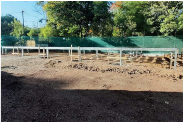
Classroom foundations being laid
