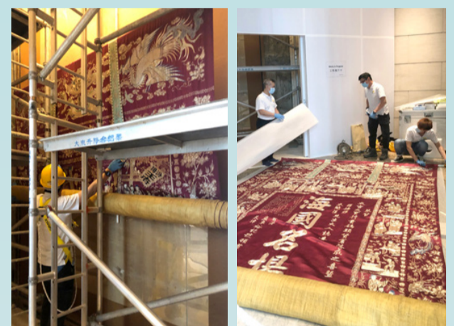
Deinstallation took place at the lobby of Cityplaza One on 31st October 2020
