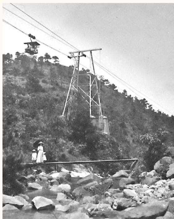
Above Contemporary image of cable car system in use with the stone foundations clearly visible.
