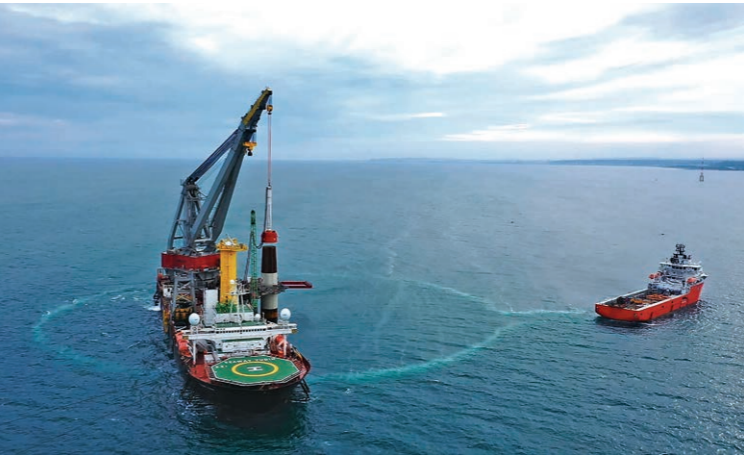
Pile driving goes ahead, with the bubble curtain deployed.
