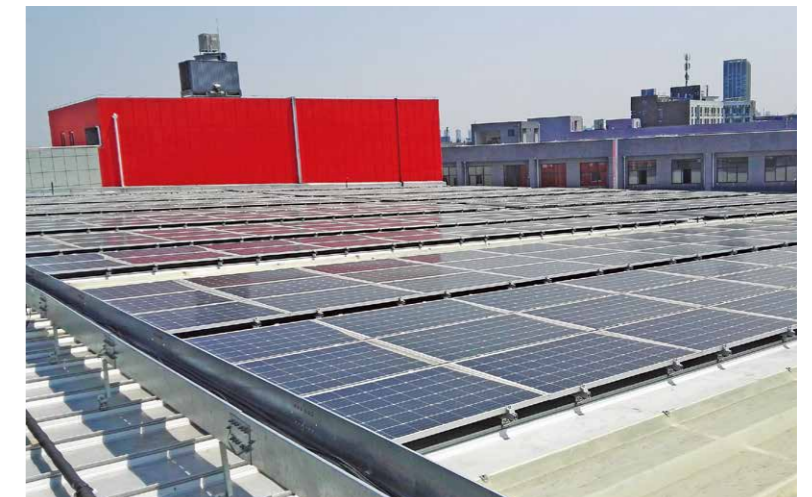
Rooftop solar panels at the Jinxiu plant have a generating capacity of 3.11 billion kWh per year.
